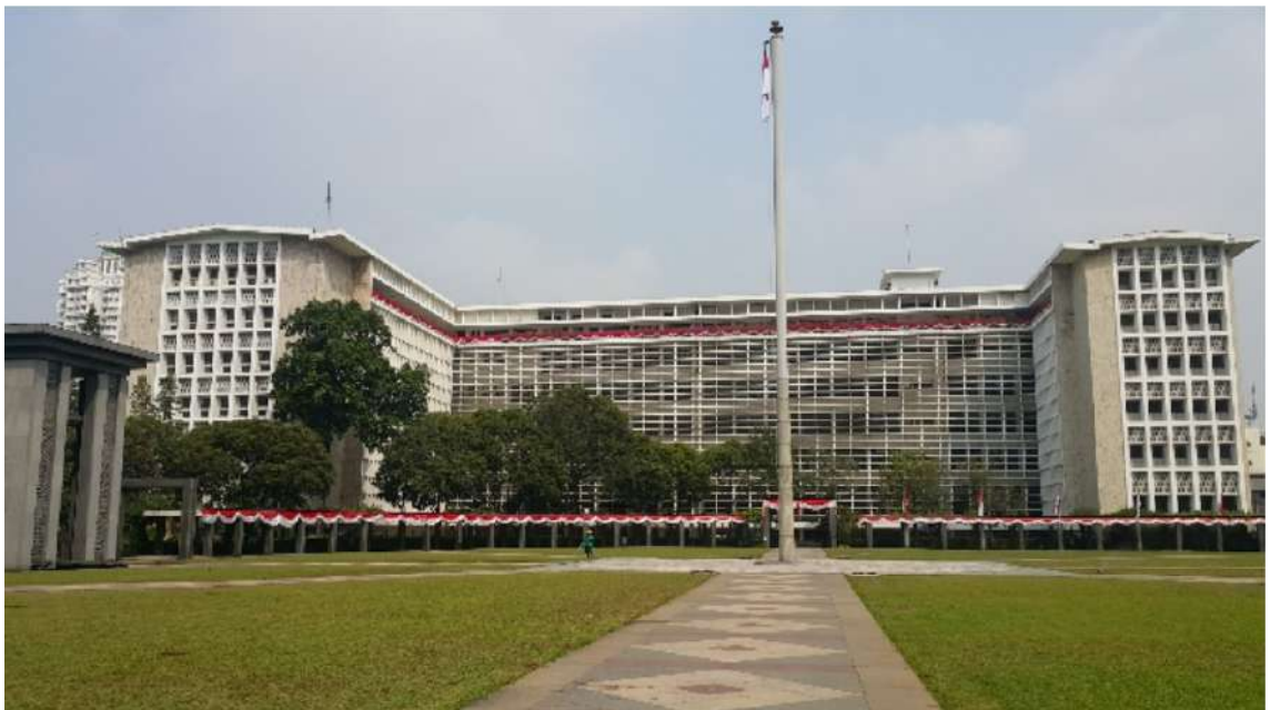
Foto 2. Tampak Muka Gedung Bank Indonesia Kebon Sirih (Survei PDA, 2018)
