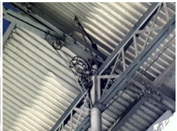
Foto 24. Detail ukiran tiang peron asli (Survei TACB 2019)
