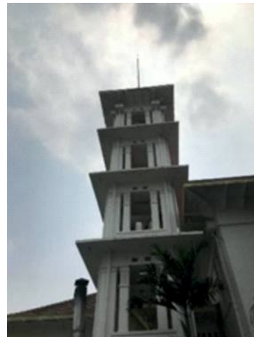
Foto 22. Base Transceiver Station Sumber: Survei TACB, 2020
