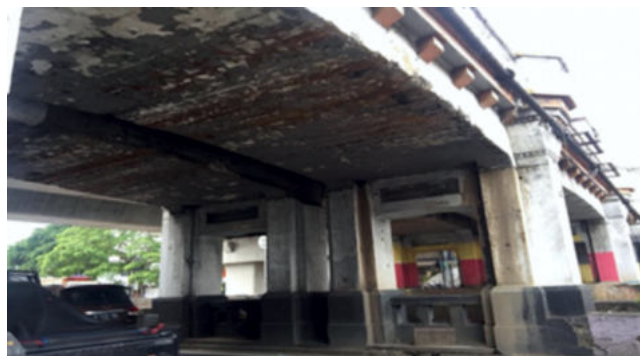
Foto 7. Detail tiang-tiang jembatan (Survei TACB 2020)
