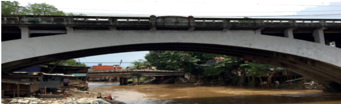
Foto 6. Detail tiang-tiang jembatan (Survei TACB 2020)
